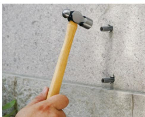
Step 5: Mount the hose hanger on the wall plugs/anchors, then insert the masonry screws into the wall plugs/anchors.
