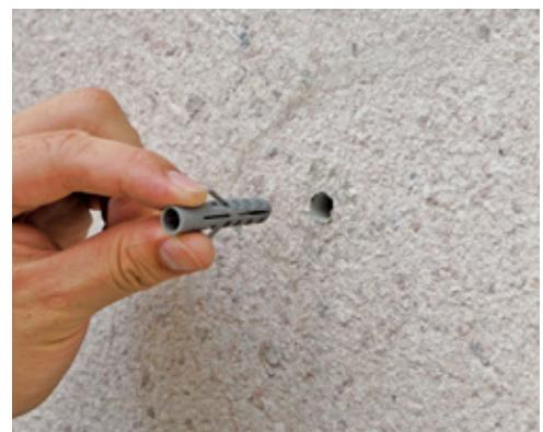
Step 4: Hammer the wall plugs/anchors into the holes.
